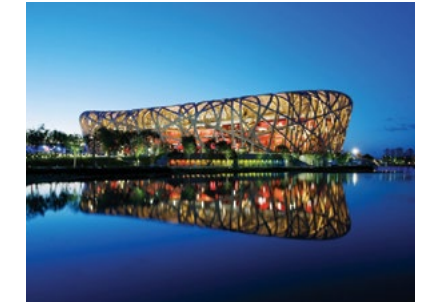
■ National Stadium (Bird's Nest)——Flame-resistance Cable
