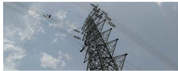
• 230kV&132kV Transmission Line for PGCB in Bangladesh
