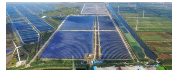
• Rudong 110 MW Photovoltaic Power Plant(BOO) in Nantong
