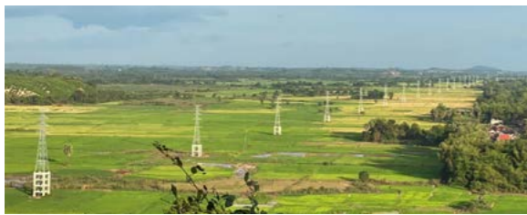
• 230kV&115kV Transmission Line for EDC in Cambodia
