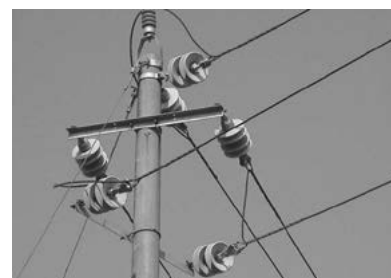
Dead-end for AAC conductor
