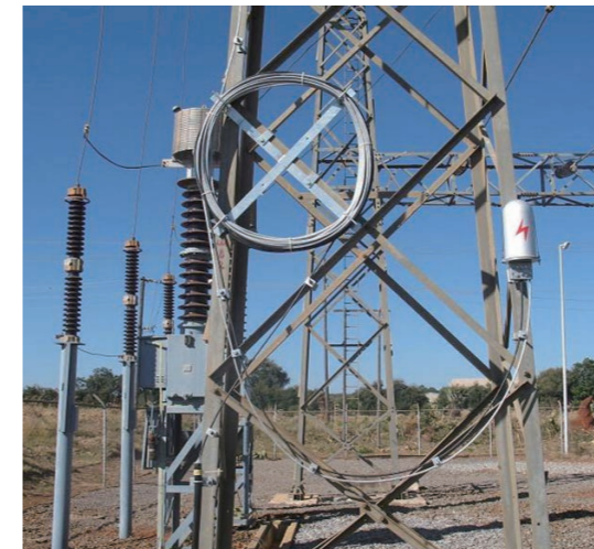
Joint box Installation
