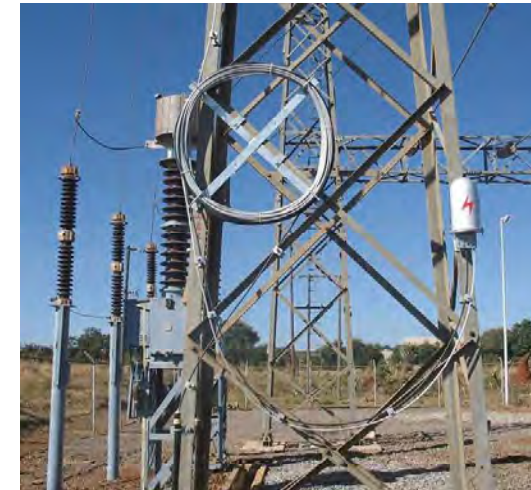
Joint box Installation
