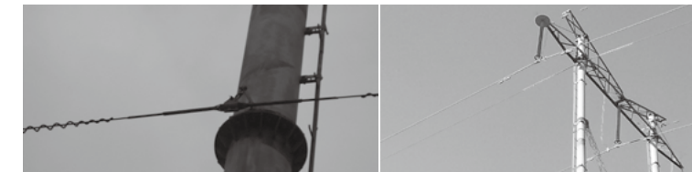
Installation on pole
