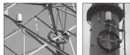
Installation on tower Installation on pole
